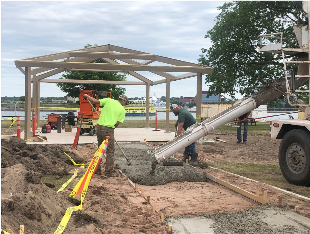
City workers placing concrete for the access ramp.
